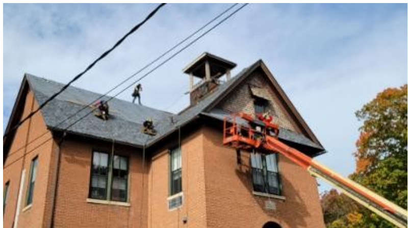
By Tuesday am, sheeting and most of the synthetic felt paper on the west side was done. South east section still had the old shingles on it. End of day saw that all shingles were removed. Please note the very hard working workers: You certainly cannot be afraid of heights
