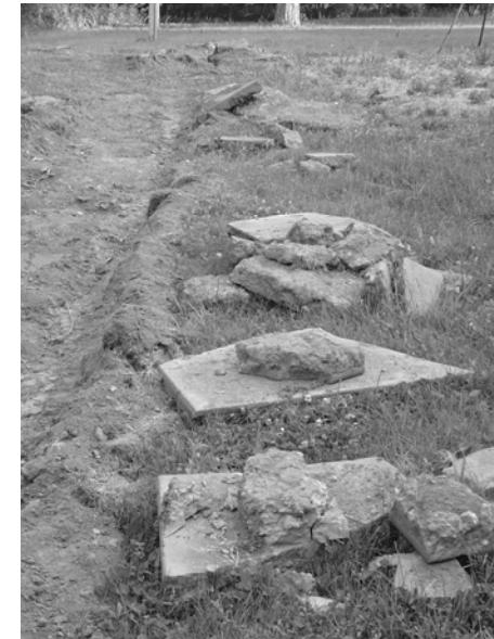
Old sidewalk is first to go.
