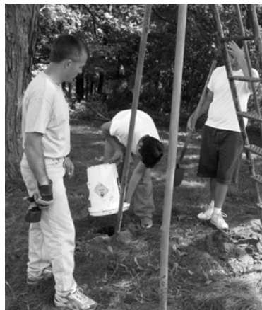
New concrete base for slide
