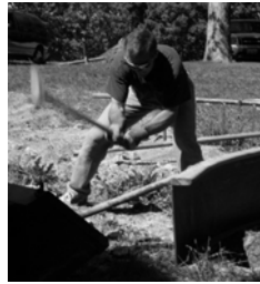
Steve removes excess concrete from slide post.
