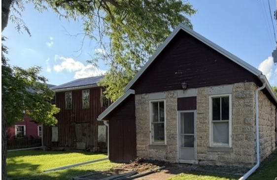
Some yard work done at the Old Jail
