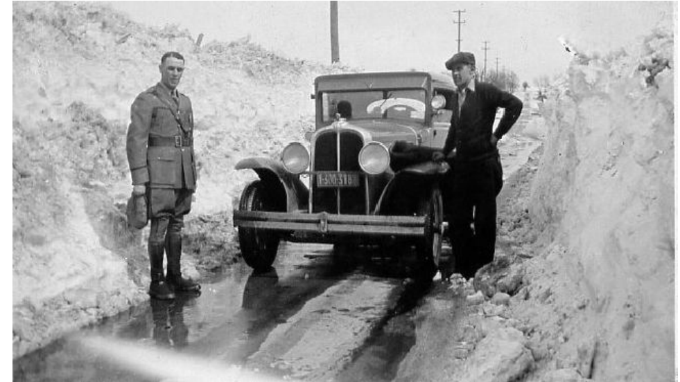
Winter storms such as those Cedarville experienced in December are nothing new to the area as proved by the photo above, probably taken between 1925 and 1929 by Merton Memler, engineer for the Il. Rt. 26 iron bridge built in 1927—28 over Cedar Creek. It has been suggested the scene is on Rt. 26 just south of Cedarville. The men and car are unidentified. Any ideas from historical society old timers?
