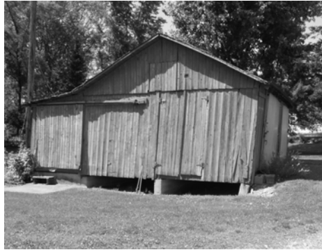
Above: South side of building
