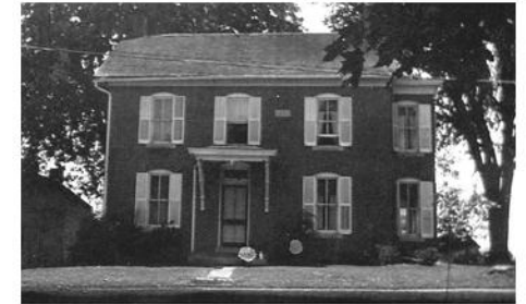
The 1888 Benson house today
