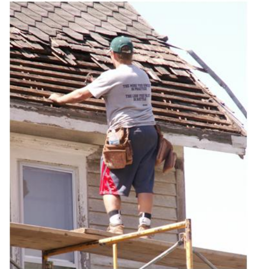
Rotting asphalt shingles and original wood shakes were removed
