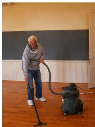
From left: Jim Bade lightly buffs first coat of floor varnish, then vacuums the dust and finally applies finish coat of varnish. Original sanding was done by Steve Myers.
