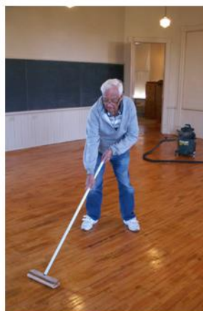
From left: Jim Bade lightly buffs first coat of floor varnish, then vacuums the dust and finally applies finish coat of varnish. Original sanding was done by Steve Myers.
