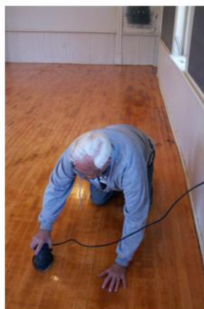
From left: Jim Bade lightly buffs first coat of floor varnish, then vacuums the dust and finally applies finish coat of varnish. Original sanding was done by Steve Myers.
