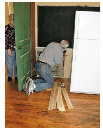
Right: Galen Bertram in last minute installation of mini-kitchen wall paneling.
