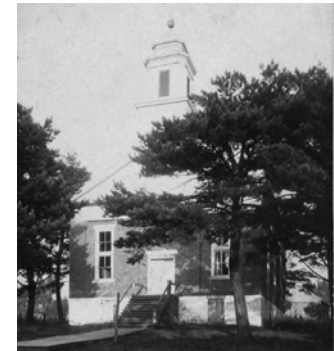
Lutheran Reformed Church built about 1853; torn down in 1960s
