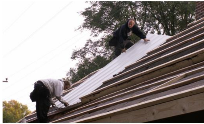
In two feverish days, the crew from Bader Construction Co., Freeport, replaced the deteriorating metal and shingle roof of the former Cedarville village jail and meeting room with a new metal roof. The historical society bought the building several years ago for $1.
