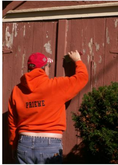
Dale Priewe works on door of attached storage room.
