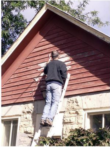
Peeling paint is removed from front by Steve Myers.
