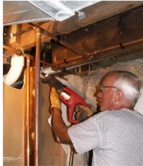
To the basement to cut a passage from there to the second floor for drainage, water and electric lines.
